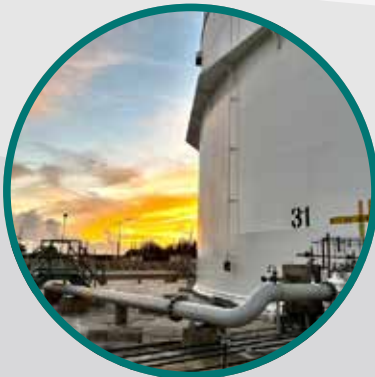
FUEL INFRASTRUCTURE REPAIR PROJECTS, WAKE ISLAND
