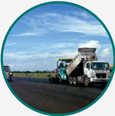
DESIGN-BUILD FAST-TRACK RUNWAY REPAIRS, BASA AIR BASE, PHILIPPINES
